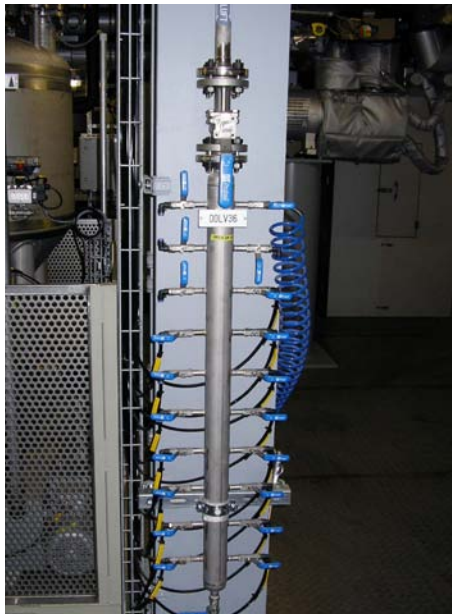
Air header INTEC with 20 outlet ports and RK-Probball Type KH2T K
