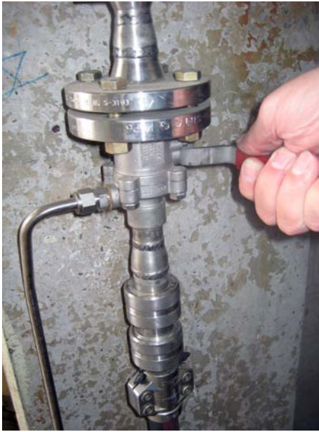
Steam ball valve INTEC K204-S-D
